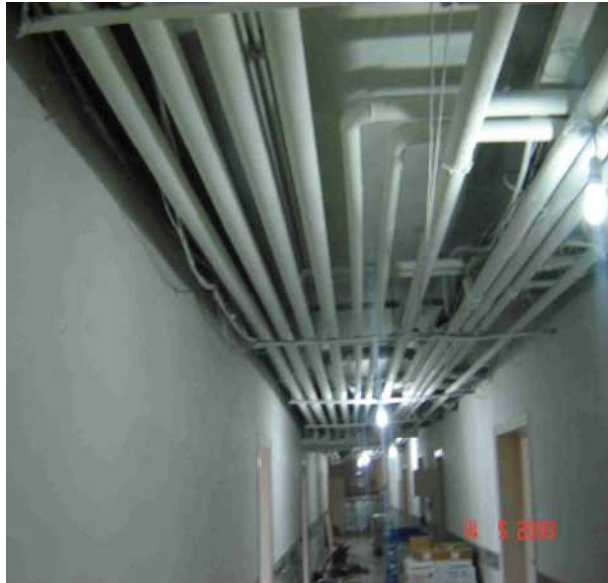
After: Insulated with MULTICERAMICS
