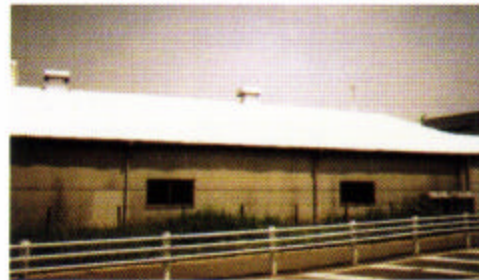
Application of SUPERTHERM
