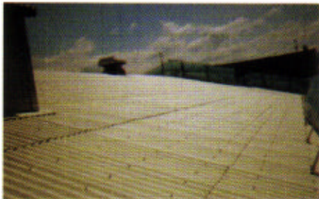
Application of SUPERBASE
